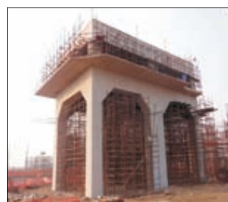
Erection work at Lime Kiln in progress at KPO
